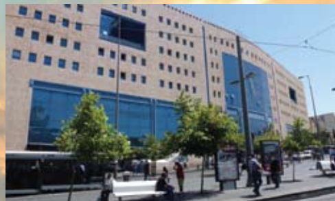
CFI's rented facilities
