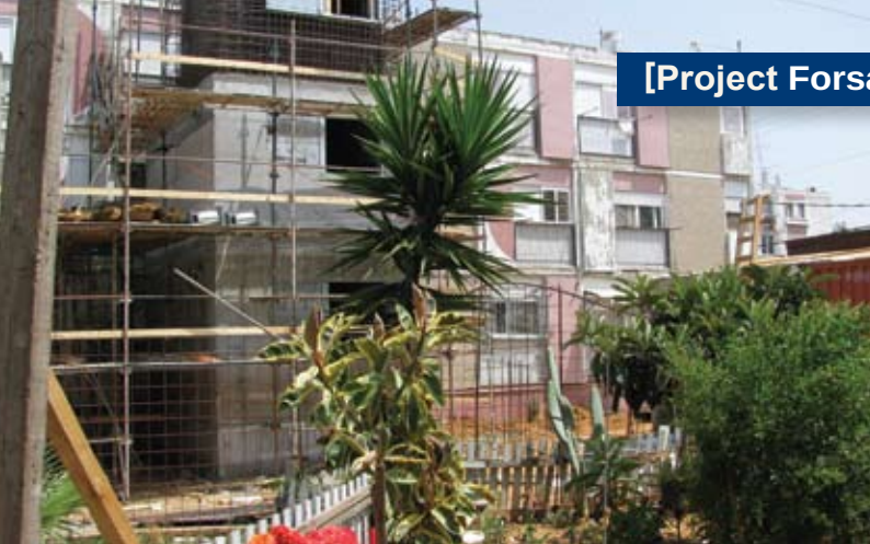
Shelter under construction
