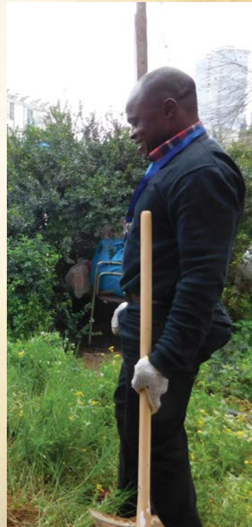
James assisting in rock removal
