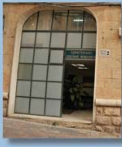
CFI former Distribution Center
